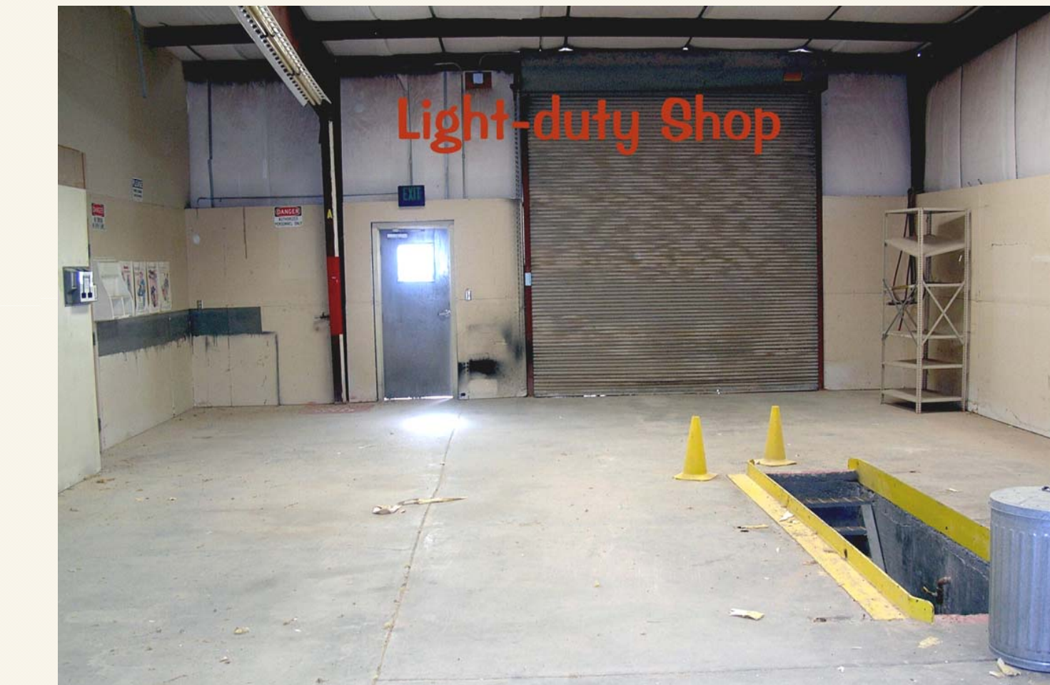
Below: Light-duty shop interior.
